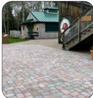
Replaced Deteriorated Bricks
